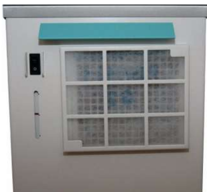
Fig. 9-11: Cooling unit filter
