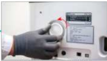
2. Pull and remove existing HEPA filters
