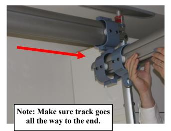
Step 22: Grab the middle track and slide the track to one end as shown in figure.
