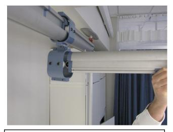
Step 19a: Grab the other end of the track and slide into the trolley.
