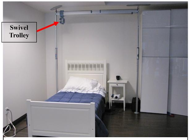
Note: Mount the adjustable track on the top pin only of the Post.
