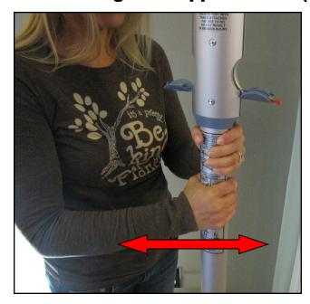
Step 8a: Grasp bottom section of post, lift slightly and adjust until bubble is centered and post is perpendicular to floor and ceiling.
