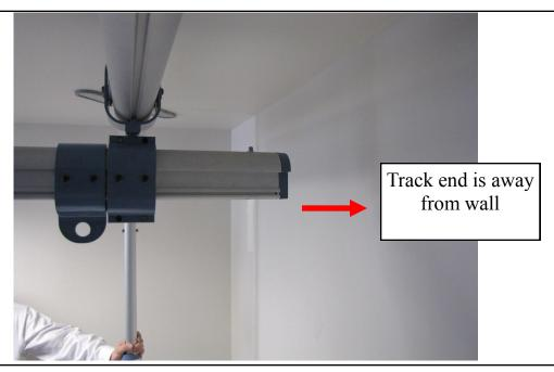
Step 24: Bring the track to the middle and make sure track end is away from the wall.
